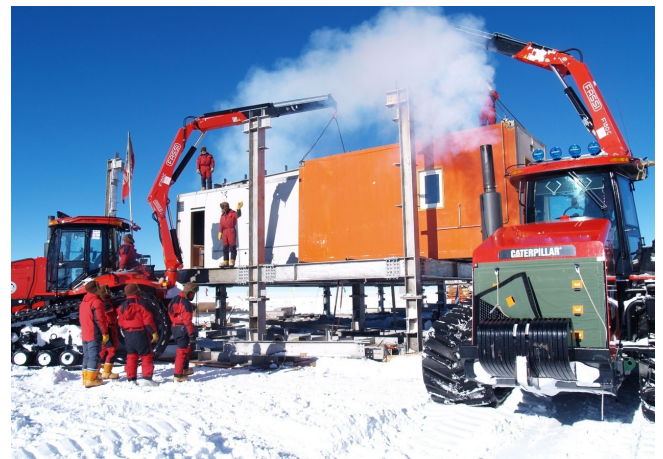
Figure 13 Hoisting the engineering cabin (Source: Chinese Arctic and Antarctic Administration, SOA).
