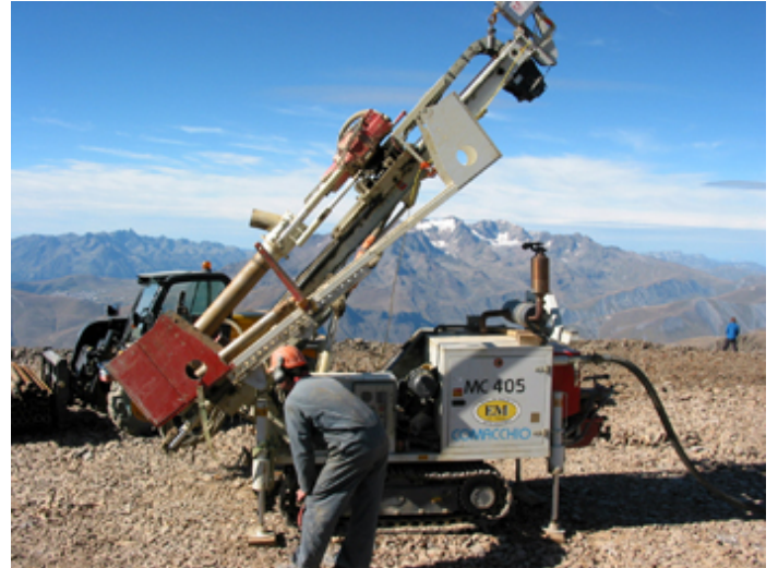
Installation of the drilling machine on the Deux Alpes observation site for the deep (100 m) borehole, at 3065 m asl. in Sept. 2010 (Photograph provided by P. Schoeneich).
