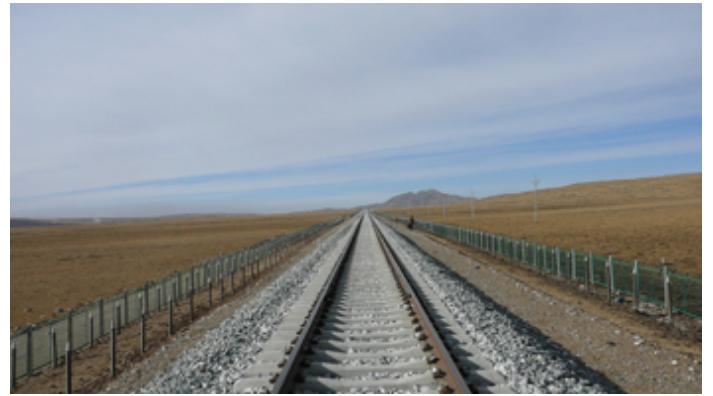
Figure 4. Air-duct ventilated blocky railbed along the Chaidar-Muli Railway
