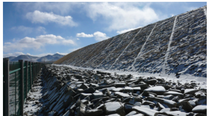
Figure 5. Side protective berm of grass mat along the Chaidar-Muli Railway
