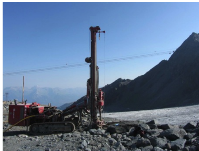
Figure 3. Drilling of a borehole in an ice-cored moraine at Col des Gentianes (Verbier, 2900 m a.s.l., Photo: C: Lambiel).
